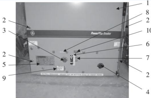
Figure 1 Front view of PowerVac breaker with front cover
